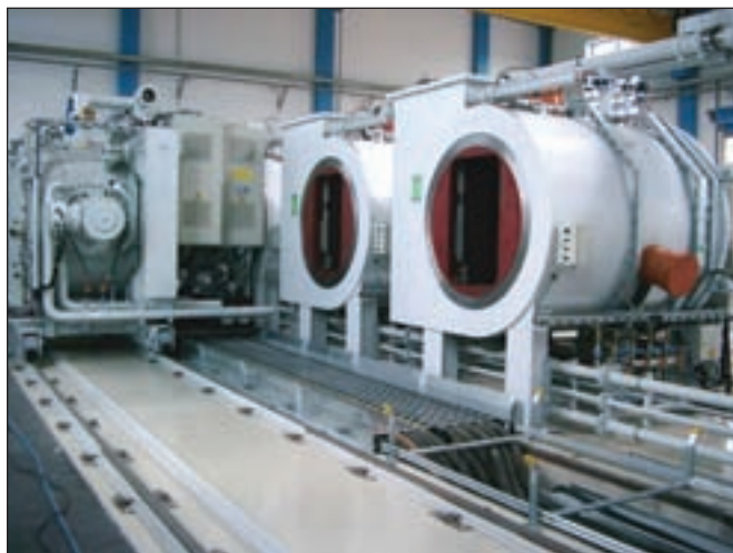
A common misconception regarding the LPC/HPGQ system seen here is increased maintenance.
